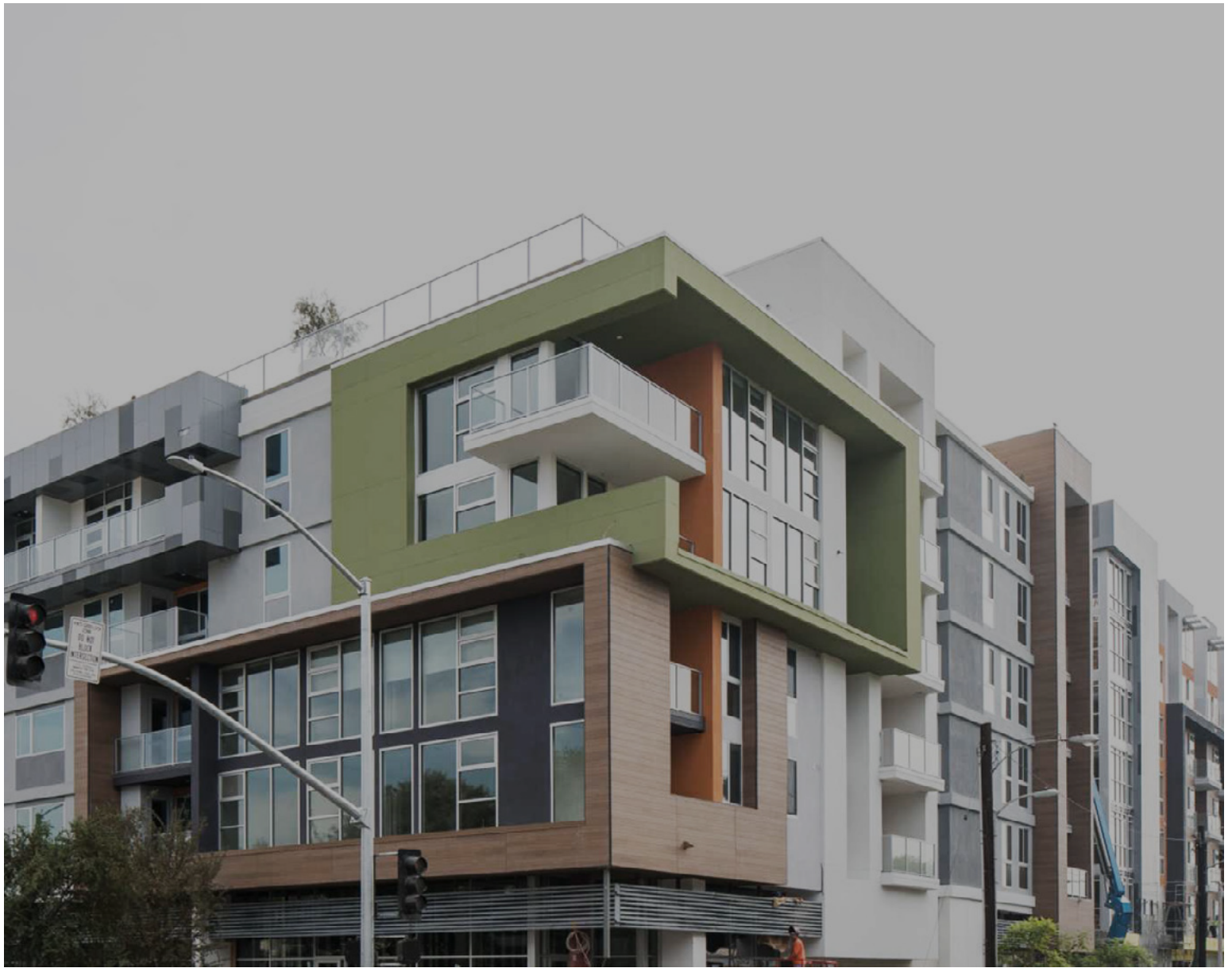
AvalonBay Communities' 668 Alameda in downtown Los Angeles will incorporate parking facilities with built-in flexibility to accommodate potential future repurposing. (AvalonBay Communities/BNIM)
