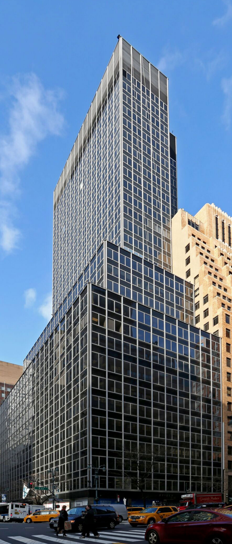
As-of-right zoning helped secure a new multifamily role for the former Pfizer headquarters in Midtown Manhattan
